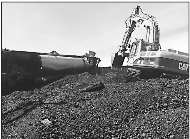
A contractor helping to clean up the derailment in Thedford. This excavator is shown on a huge pile of coal that was spilled in the derailment.
