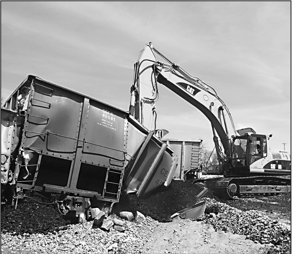
An excavator picks up and moves a wrecked coal car, before beginning the work of cleaning up the spilled coal.
