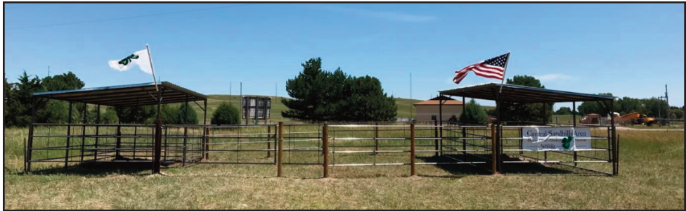
The new Thomas County 4-H livestock facility at the fairgrounds near Thedford.
